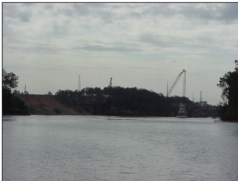
Photo 1. Bernard Bayou at Entrance to Industrial Seaway
